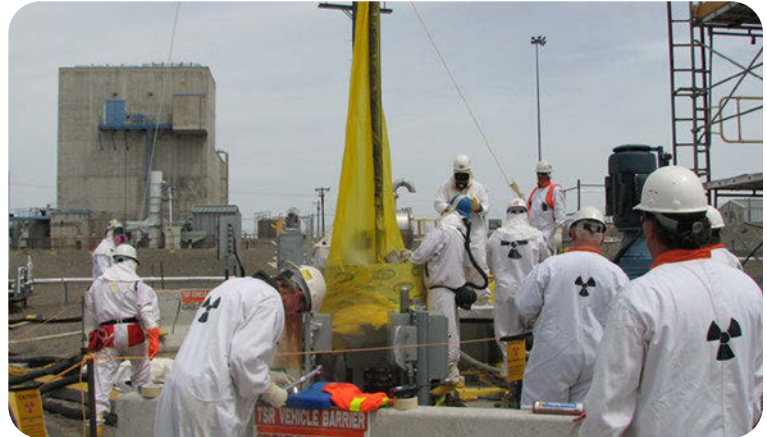
Crews pump waste from single-shell tanks at the Hanford Site to more stable double-shell tanks. (Photo: DOE)
