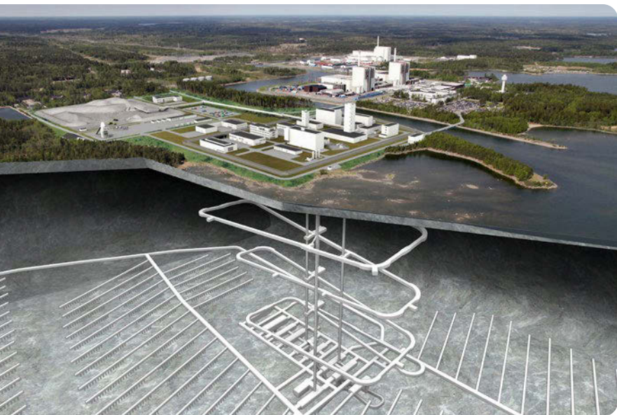
Rendering of the Forsmark geologic repository for spent nuclear fuel in Sweden. Below ground, the repository covers three to four square kilometers at a depth of 500 meters. (Image: SKB)
