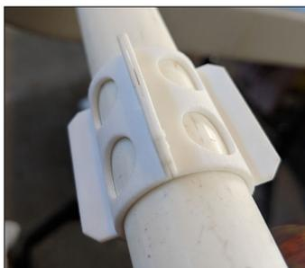
**Figure 14. Centralizer on ¾-inch [1.9 cm] PVC conveyance pipe during grouting.**
